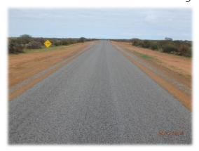
15.2 km two-coat, 7.2m wide seal including floodway stabilisation completed at the southern boundary of the Shire. A 1.0km section around Curbur has also been completed. As outlined elsewhere in this issue, a great effort from all.
