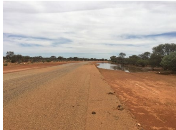
Road level causing ponding on one side.
