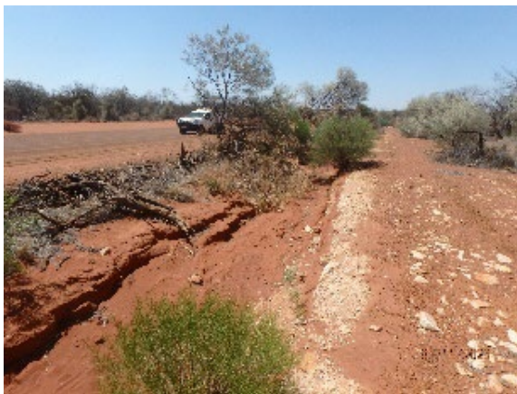
New road but old road formation still retained causing scouring and retention of floodwaters.
